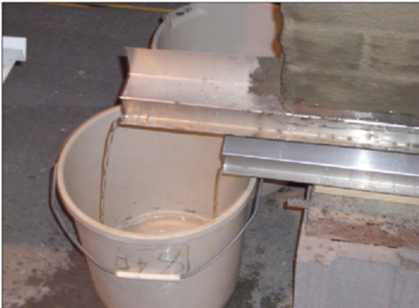
Loxon Panel Drainage (Photo 4)
