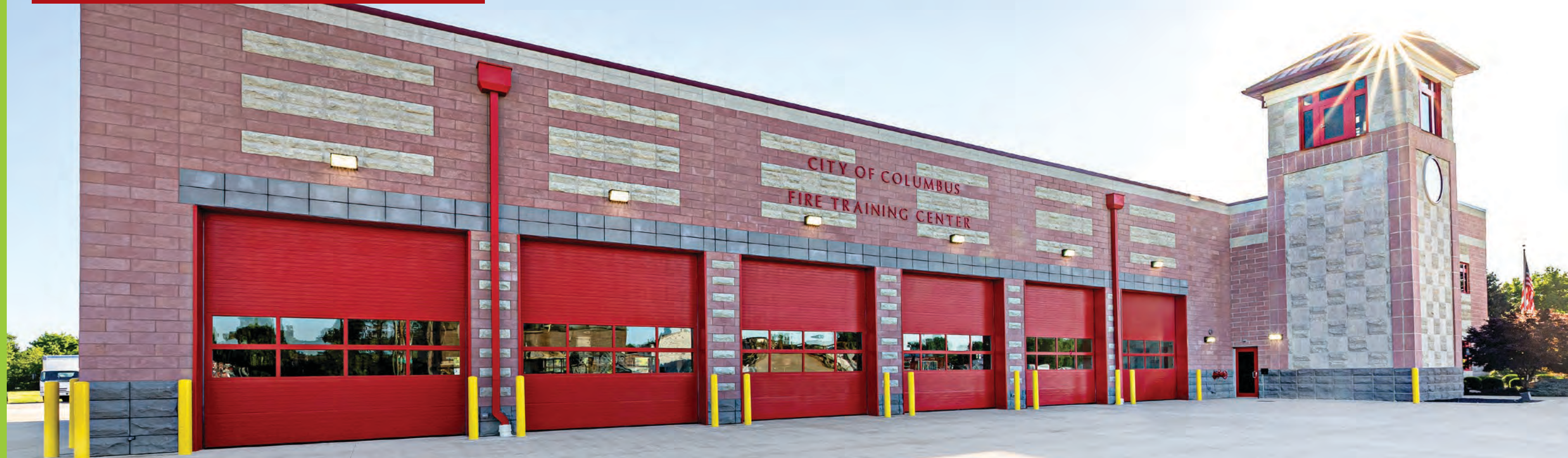
Columbus Fire Department – Training Academy Building | HKI Associates | ARRIS-clip Custom
