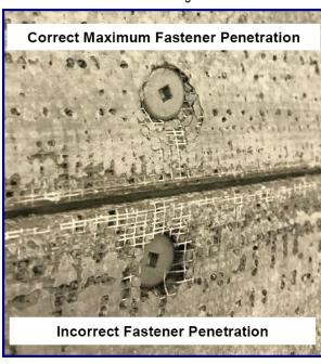
Engineer of Record should select screws and screw spacing using <u>NTA Report TRIG030116-28</u>. Screw spacing will be dependent on weight of the thin adhered masonry veneer or synthetic stucco application, insulation thickness, wall height, wind pressure, wind speed, and whether the installation is a **supported** or **unsupported** panel application.
