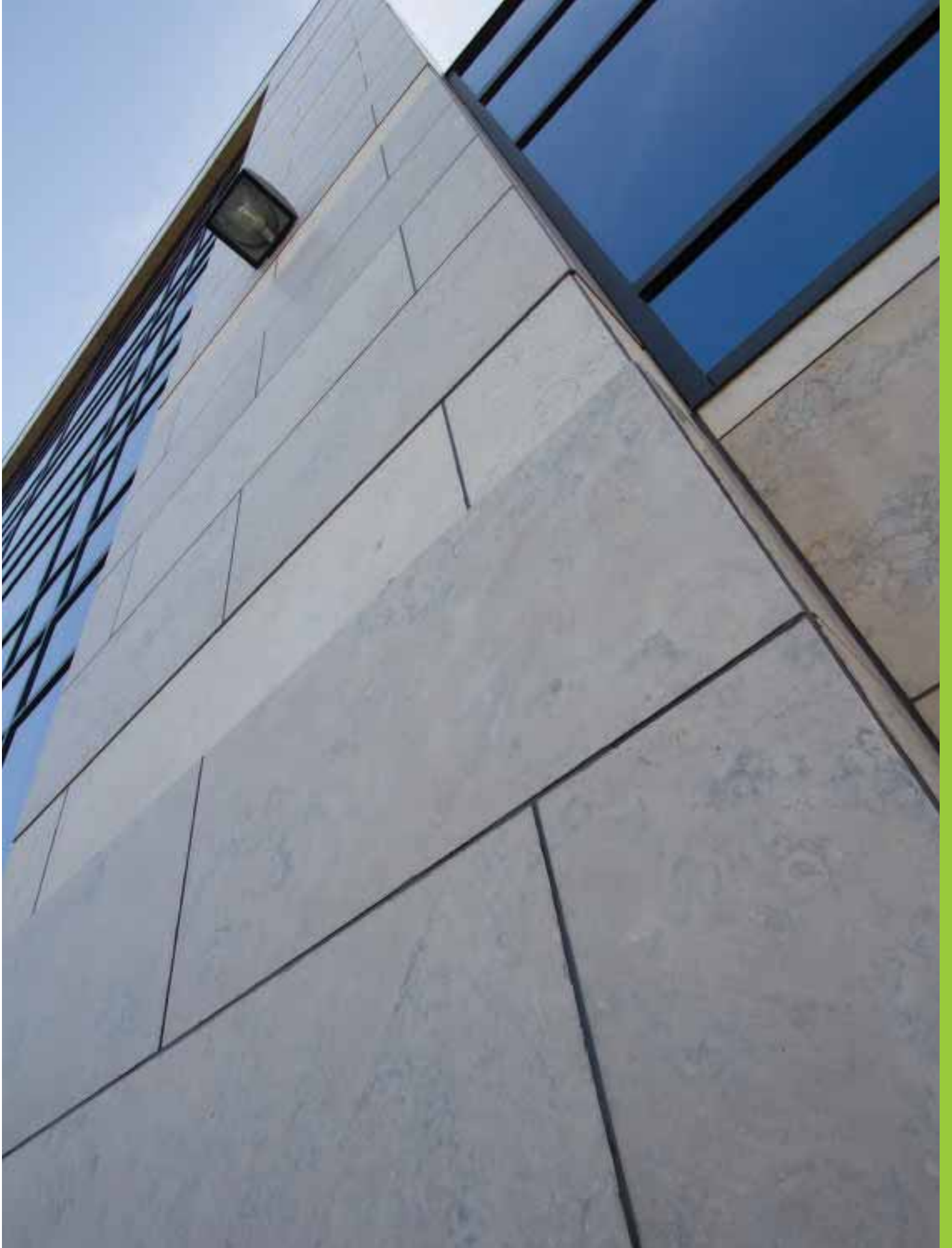
Commerce Court Office Building | A Baldassarra Architect Inc. | Adair® Sepia Fleuri
