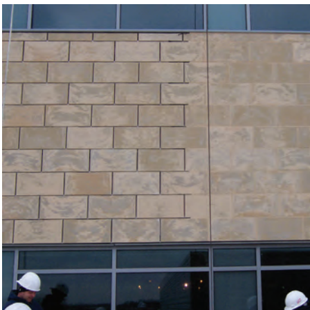
Step 7: Joints Sealed with Backer Rod and Silicone Sealant
