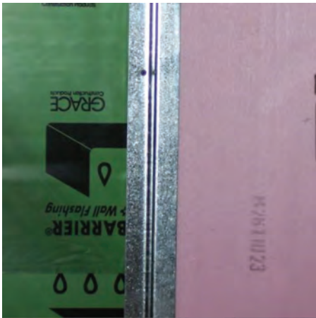
Step 4: Install "Z" channels and then Rigid Insulation between "Z" channels
