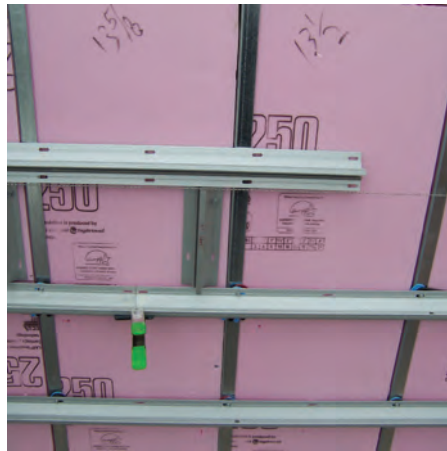
Step 5: Install Gridworx Channels over "Z" channels and rigid insulation
