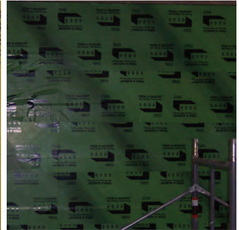
Step 3: Waterproofing Membrane
