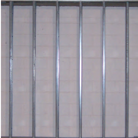
Step 1: Steel Studs
