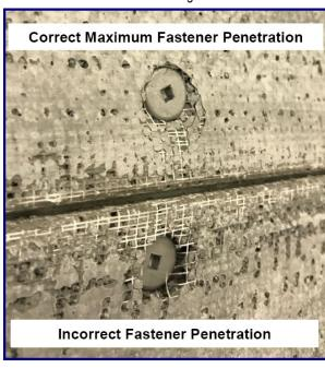
Engineer of Record should select screws and screw spacing using <u>NTA Report TRIG030116-28</u>. Screw spacing will be dependent on weight of the thin adhered masonry veneer or synthetic stucco application, insulation thickness, wall height, wind pressure, wind speed, and whether the installation is a **supported** or **unsupported** panel application.
