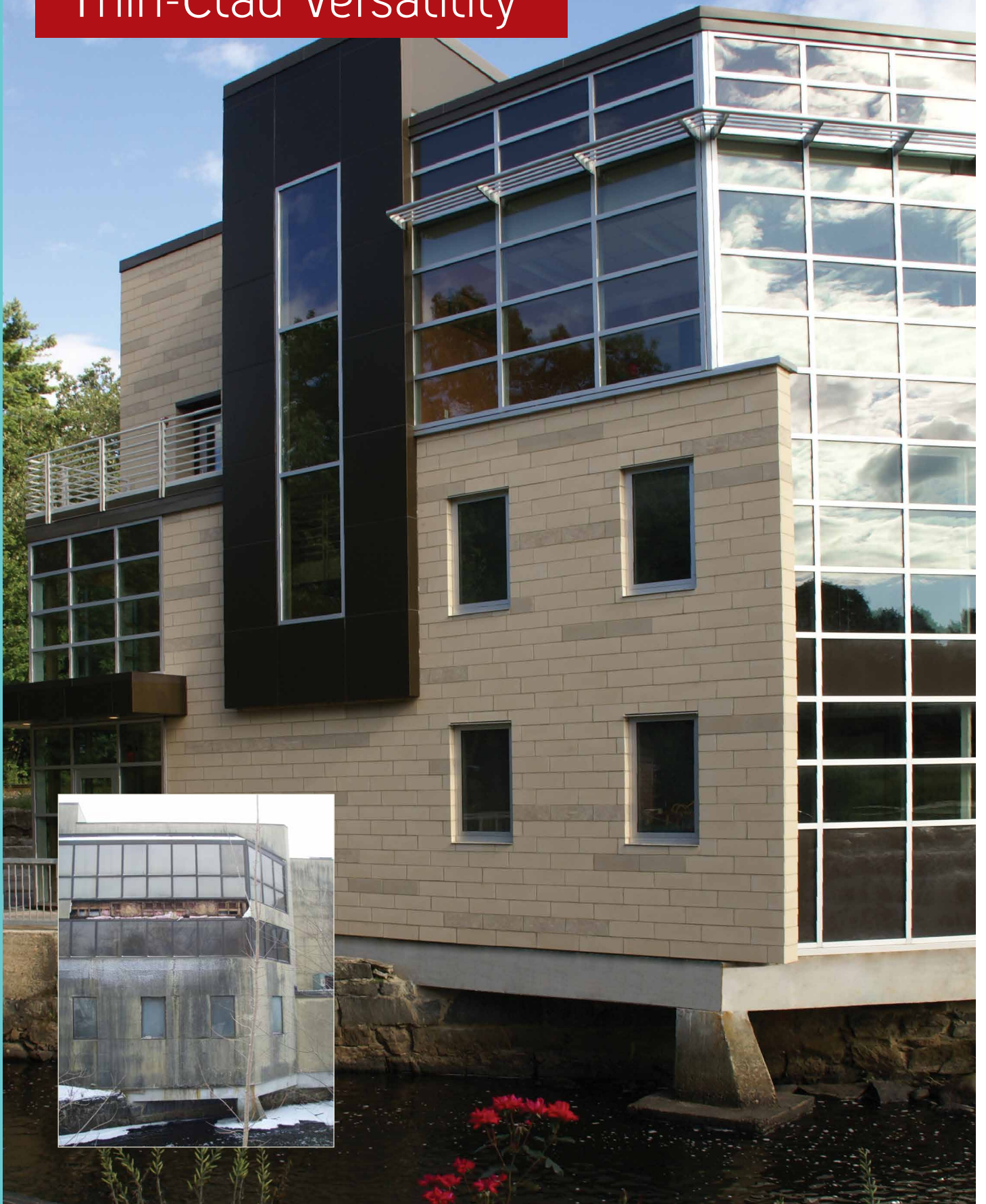
P&S Office Building | North Chelmsford, MA | Design/Build by P&S Construction | ARRIS-clip exterior, ARRIS-tile interior
