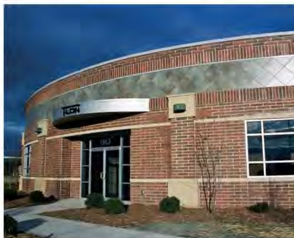
Single Wythe Half-High Construction in Hartland, Wisconsin
