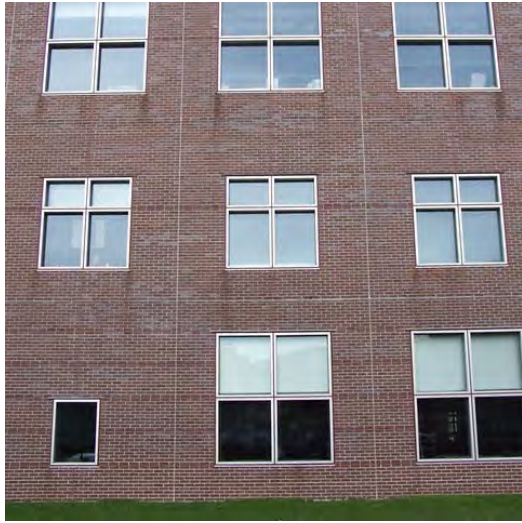
Figure 12: Placement of movement joints creates wall symmetry.
