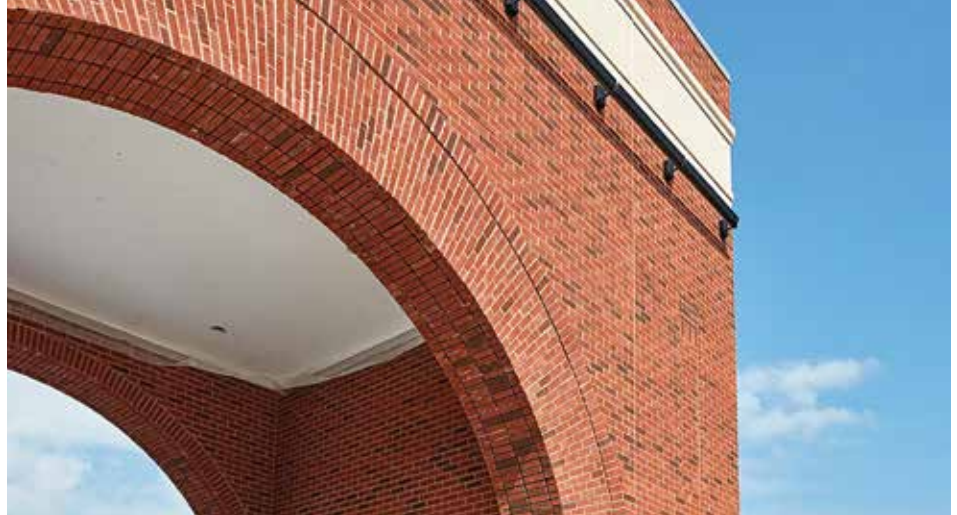
NEW ETSU STADIUM
