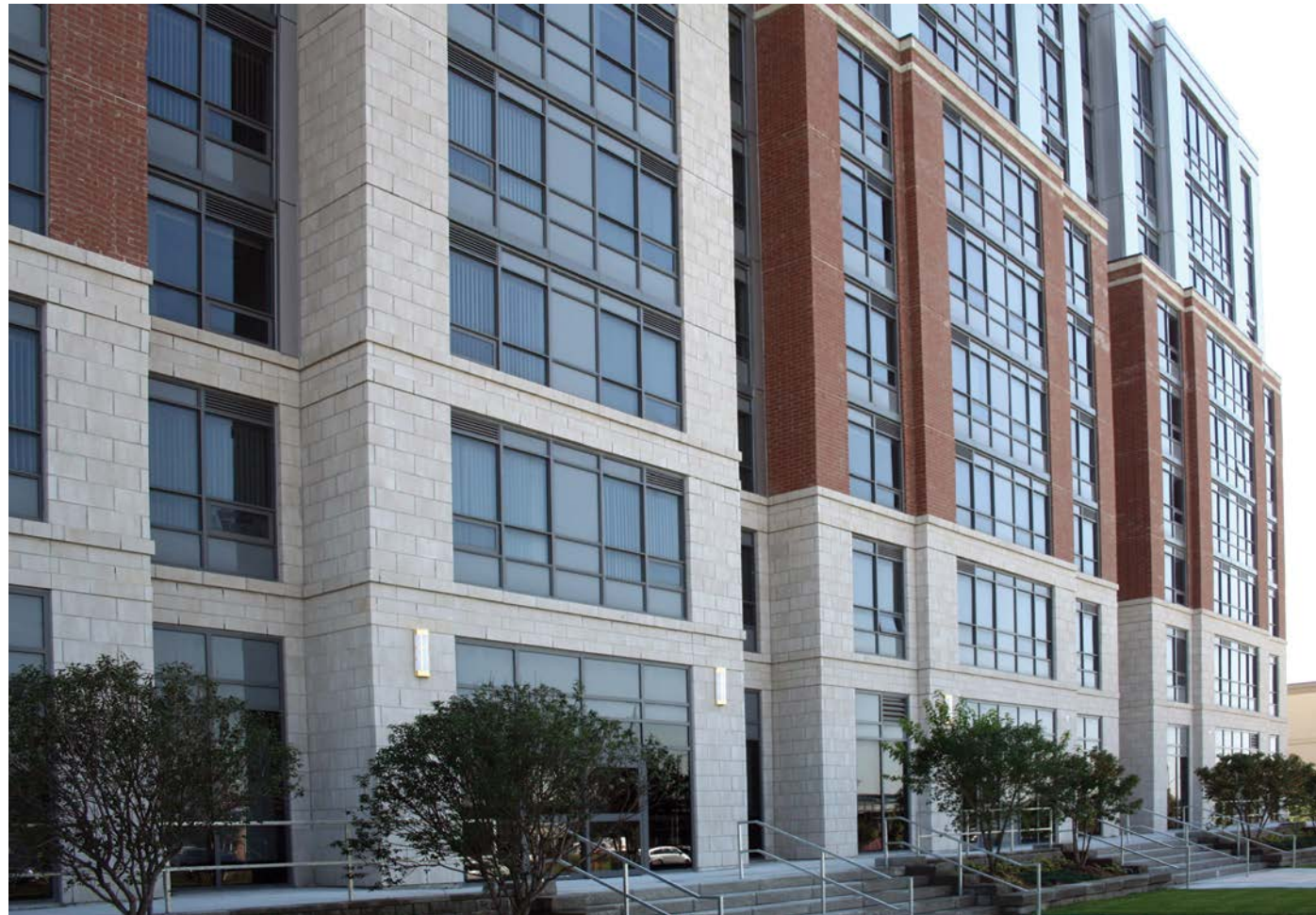
Mon Sheong Court, Richmond Hill, ON | Burka Architect | Muscade Jet de Sable
