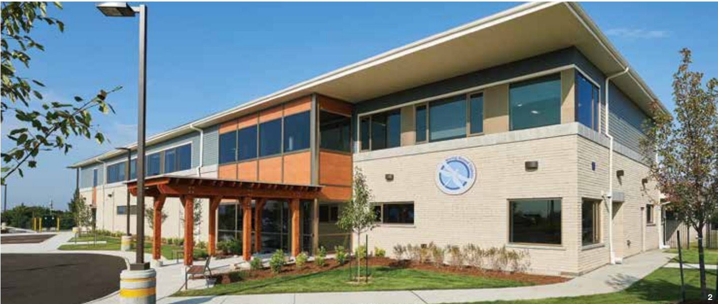
1. Ray & Tye Noorda Oral Health Sciences Building, University of Utah School of Dentistry; MHTN Architects, Color: Custom | 2. Haven House, Cambridge, ON; MMMC Architects; Color: Ivory White
