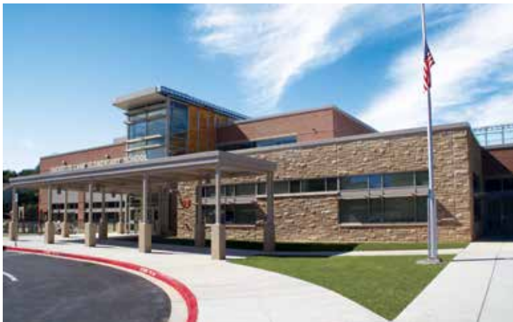
Ducketts Lane Elementary School; Grimm + Parker Architects; Color: Custom
