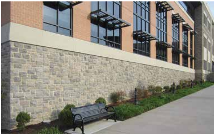
Richmond Hill Montessori and Elementary Private School; IBI Architects; Color: Algonquin custom blend
