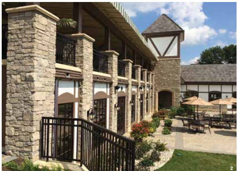
1. The Lion's Gate at Penn State Abington, Abington, PA; SMP Architects; Color: Twilight | 2. Kenwood Country Club, Cincinnati, OH ; Color: Eclipse
