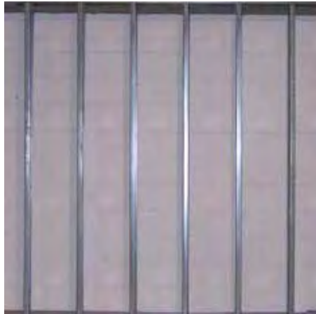
Step 1: Steel Studs
