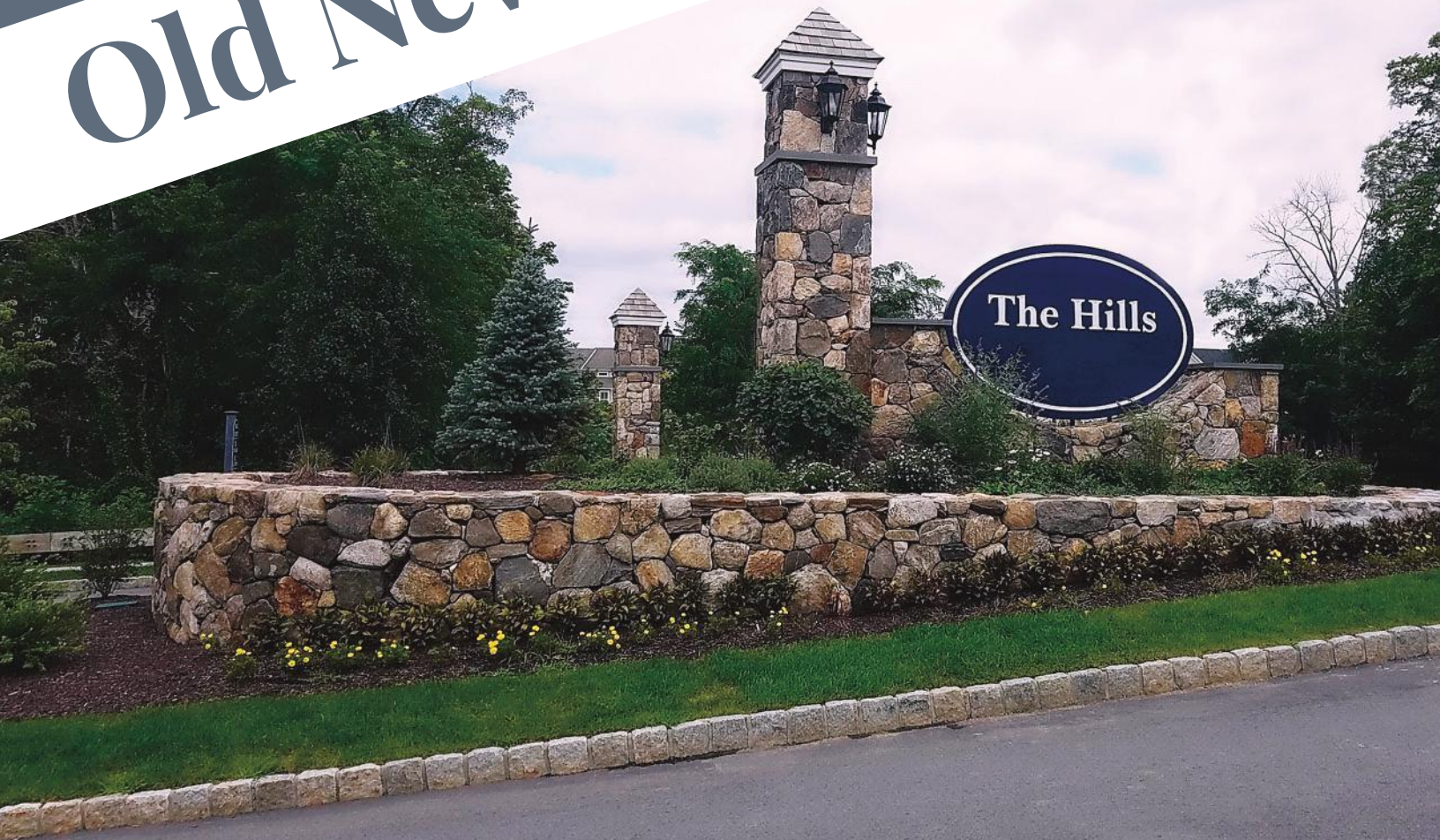
Photo: Toll Brothers (CT)
