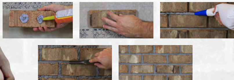
Interior Adhesive Installation
