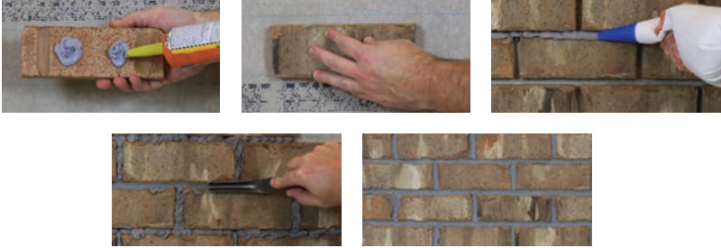
Interior Adhesive Installation
