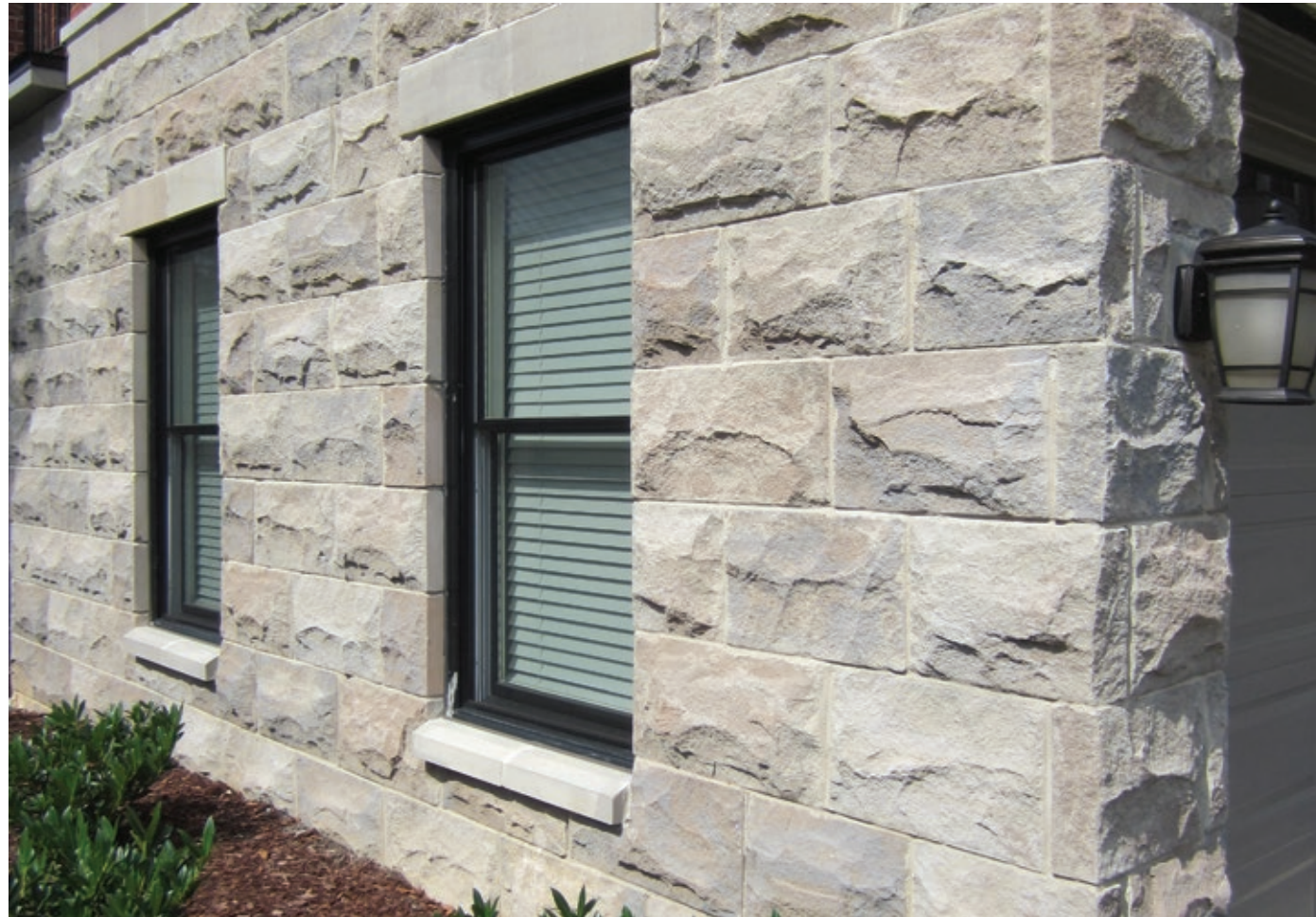
The Court at Lyon Village - Arlington, VA | W. C. Ralston Architects | Driftwood Rocked and Sandblasted
