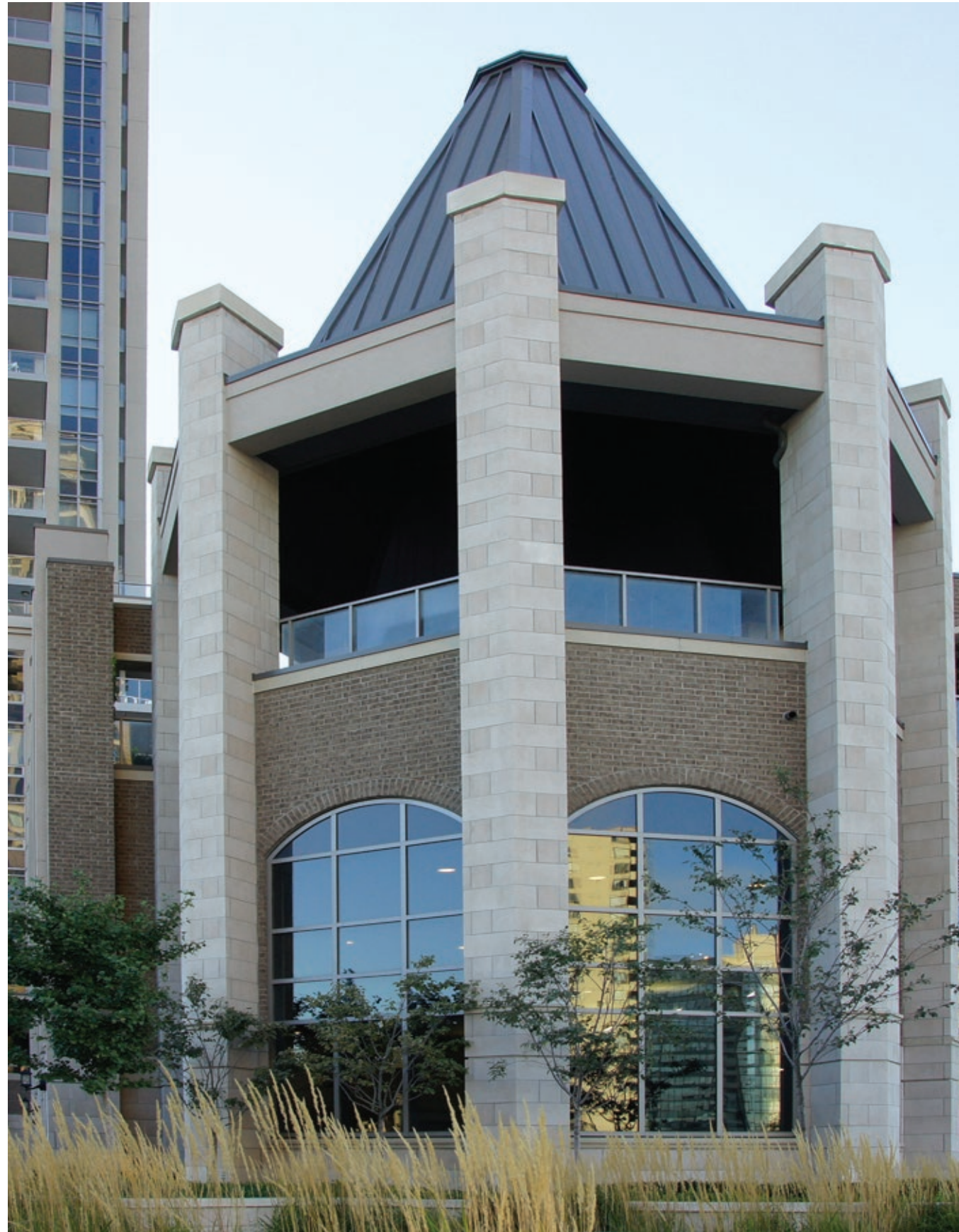
388 Prince of Wales Dr. - Mississauga, ON | Kirkor Architects | Nutmeg Sandblasted
