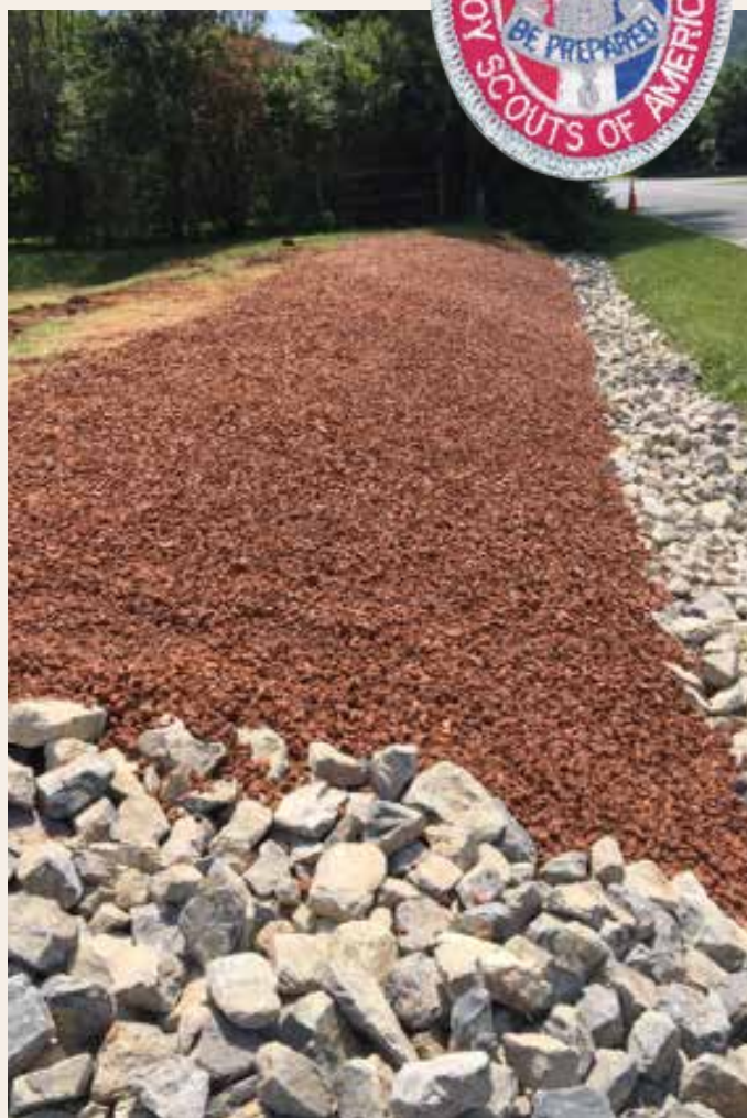
General Shale donated 20 tons of brick chips for the project.
