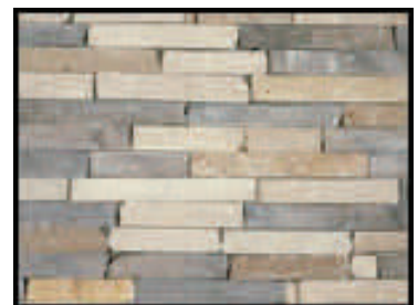
No Mortar Joint (Dry-Stacked)
