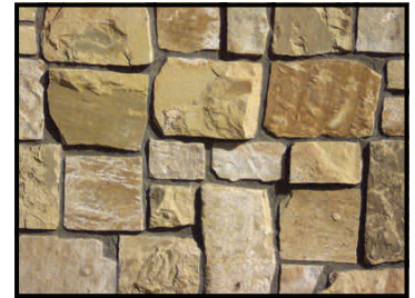
Standard 1/2" Mortar Joint
