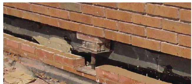
Photo 4 Flashing Installation Using Temporary Support
