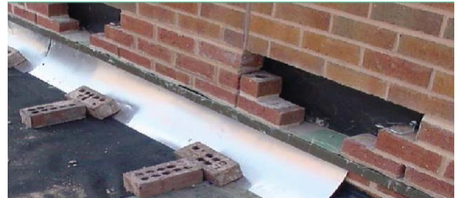
Photo 3 Flashing Installed in Alternating Sections
