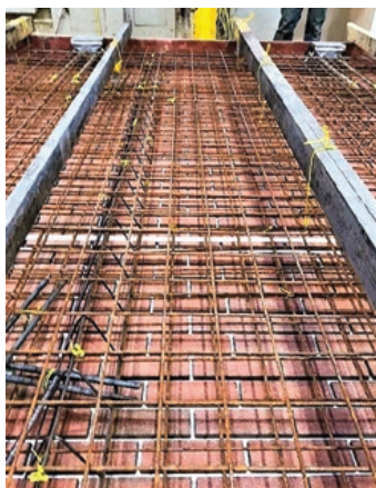
Thin brick installed in form liner
