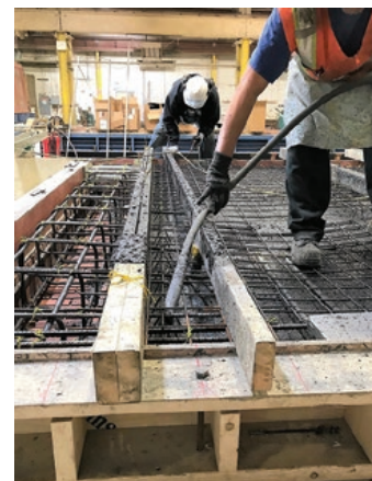
Concrete being vibrated in place
