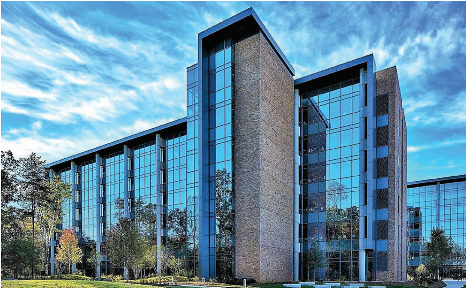
LPL Financial Eastern Headquarters | Fort Mill, SC | Architectural Classics | Old Monobuck (tumbled)
