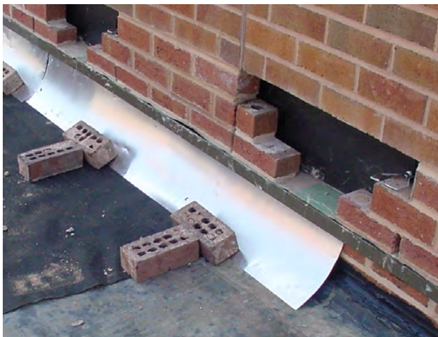
Photo 3 Flashing Installed in Alternating Sections
