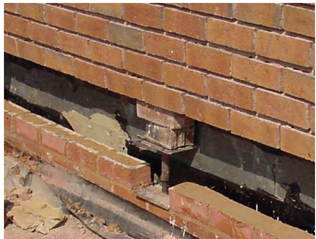
Photo 4 Flashing Installation Using Temporary Support
