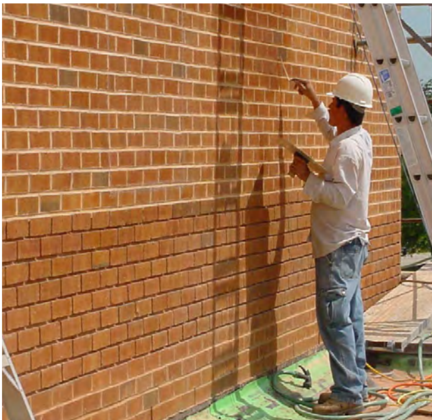
Photo 2 Repointing Mortar Joints
